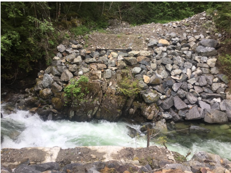
Left Bank Abutment when facing downstream
